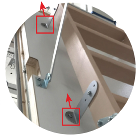
Ladder mounted higher up on the trapdoor.
